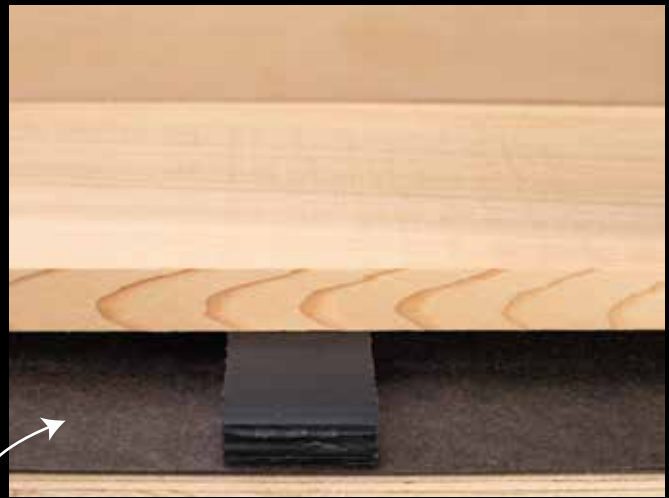
Cor A Vent Plastic Furring Strips Over 2 Ply Felt Paper
