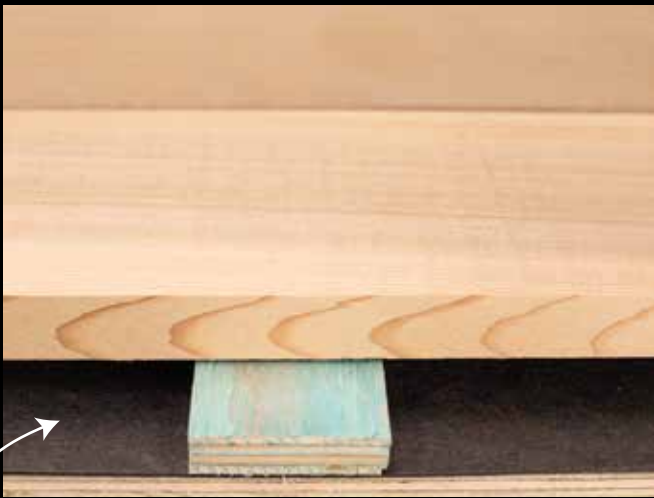
Treated Plywood Furring Strips Over 2 Ply Felt Paper
